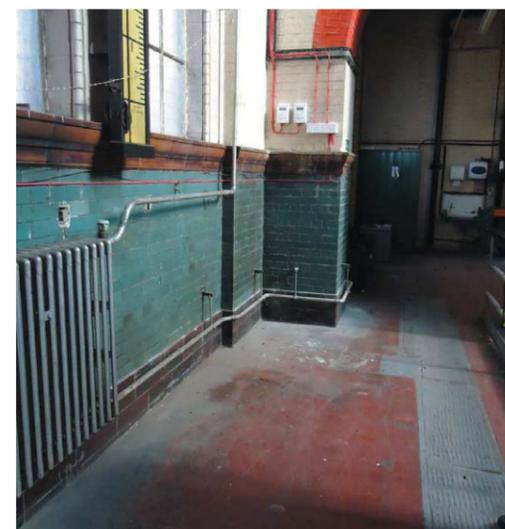
Figure 14.33: Example of glazed brick inside pumping station - location 'B'
