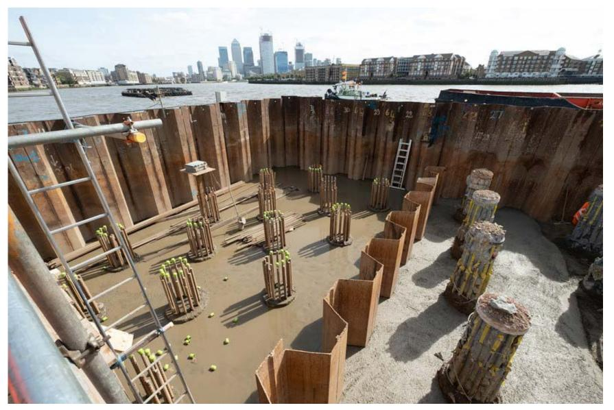
Piles are broken down ready for concrete slab and concrete beams
