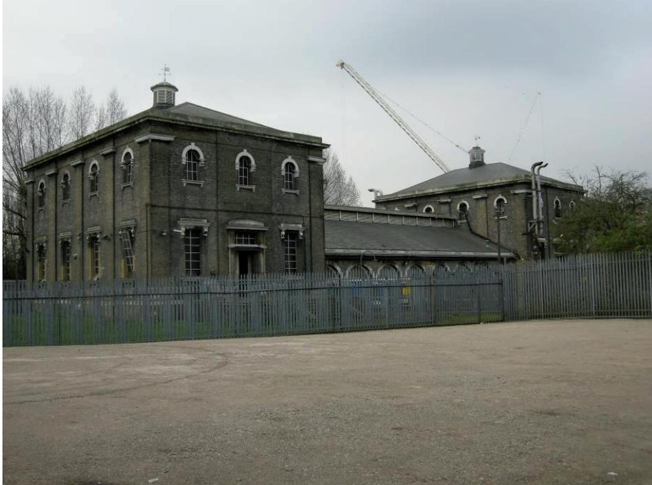
**Vol 24 Plate E.10 Historic environment – The northernmost of the two Grade II listed coal sheds (HEA 1B and 1C) in the southwestern part of the site. The cast iron columns are hollow and function as drainpipes; standard lens, looking southeast**
