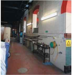
Figure 14.32: Preferred location for electrical and control equipment inside pumping station - location 'A'
