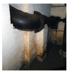
Figure 14.31: Cast iron gas main to be removed to accommodate ducting
