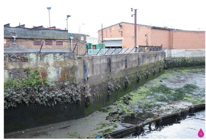
Figure 10.3: Floodwall of Bell Lane Creek
