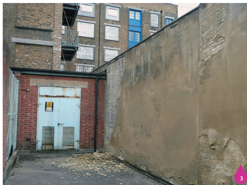
Figure 21.6: Existing switch gear and transformers
