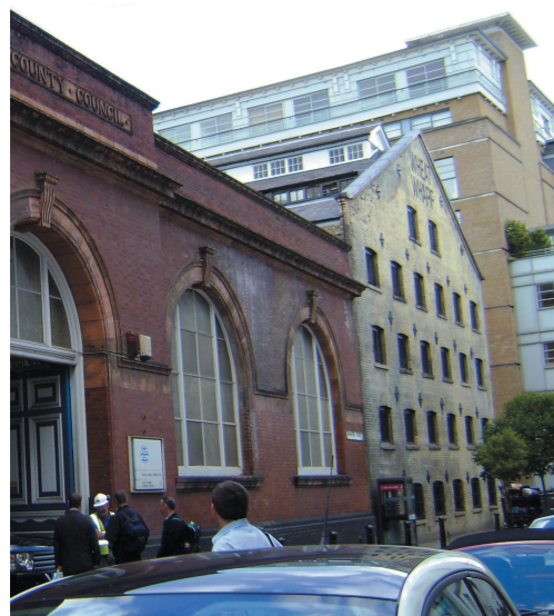
Figure 21.33: Existing front entrance and side door
