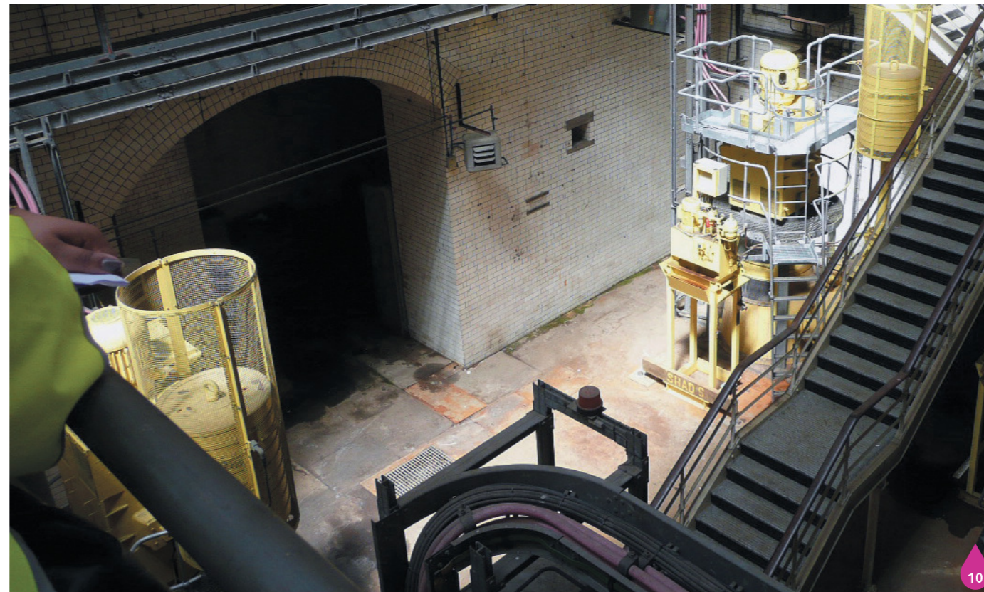
Figure 21.18: View inside pumping station
