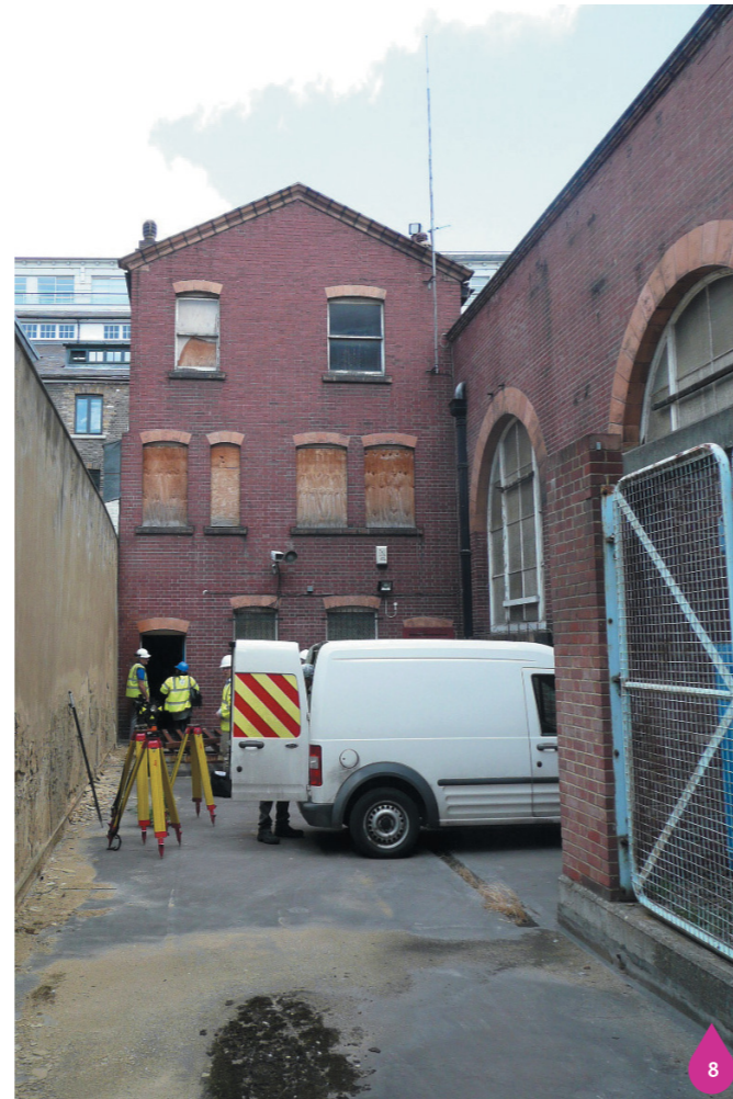
Figure 21.16: View of the facilities building from within courtyard
