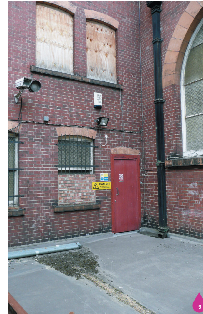
Figure 21.17: View within pumping station courtyard
