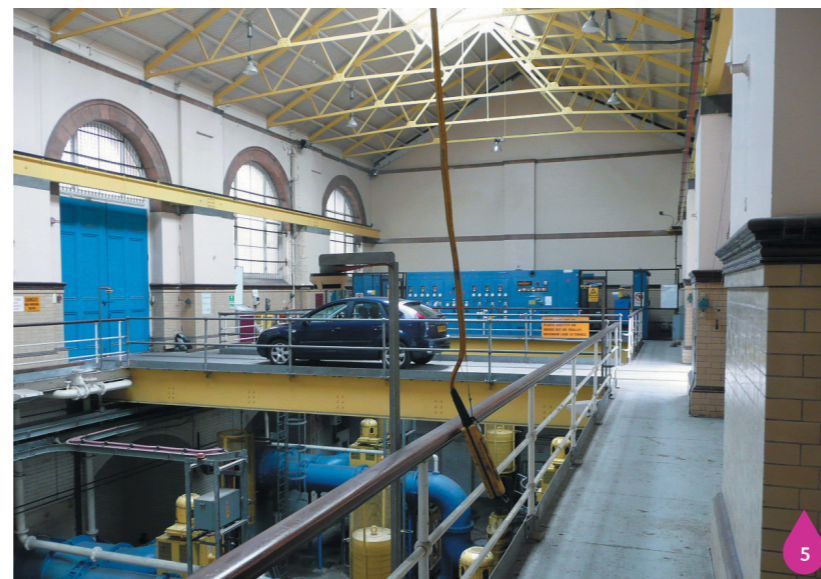
Figure 21.8: View inside pumping station
