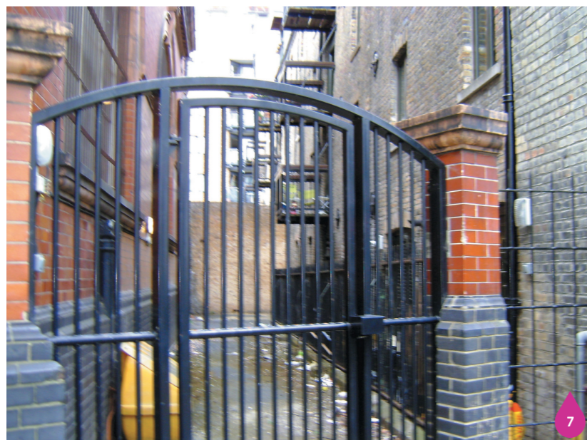
Figure 21.15: Side gate pedestrian entrance
