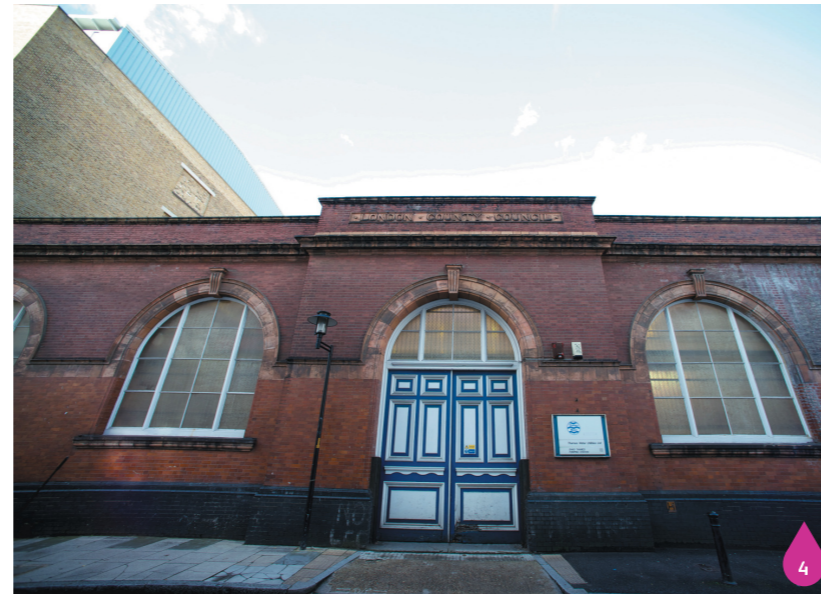
Figure 21.7: Front door of main pumping station
