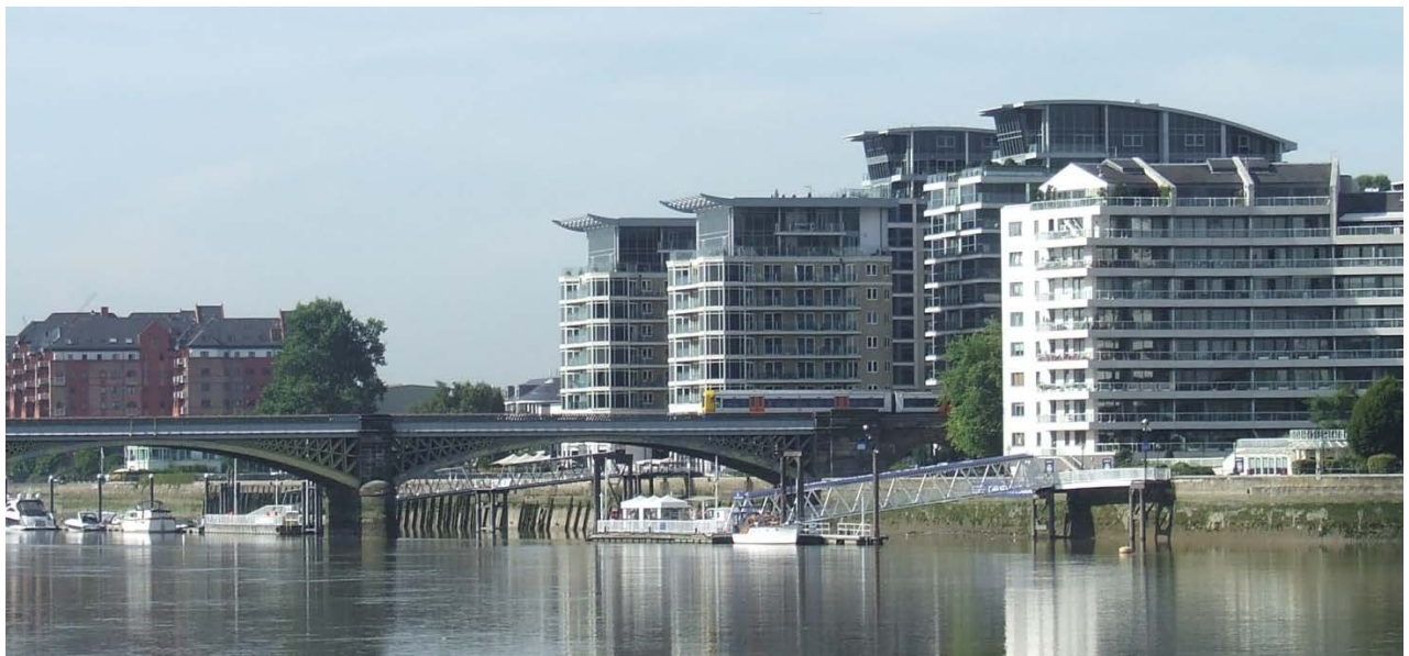
Figure 7.2 Chelsea Harbour Pier
