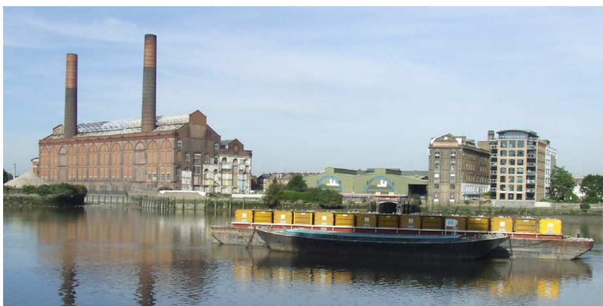
Figure 5.1 Lots Road Power Station and Cremorne Wharf
