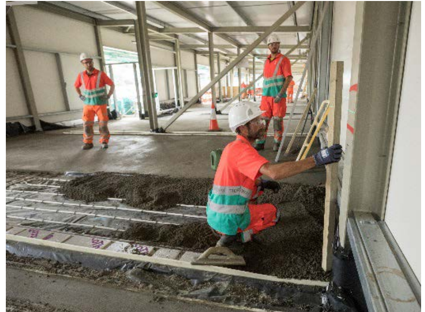
Screed Flooring & Internal Drainage
