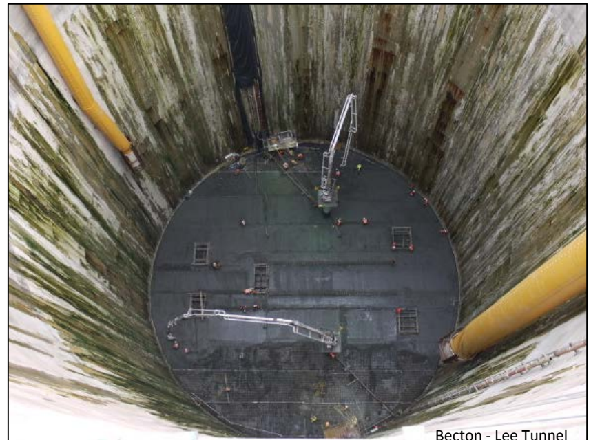
Becton - Lee Tunnel
