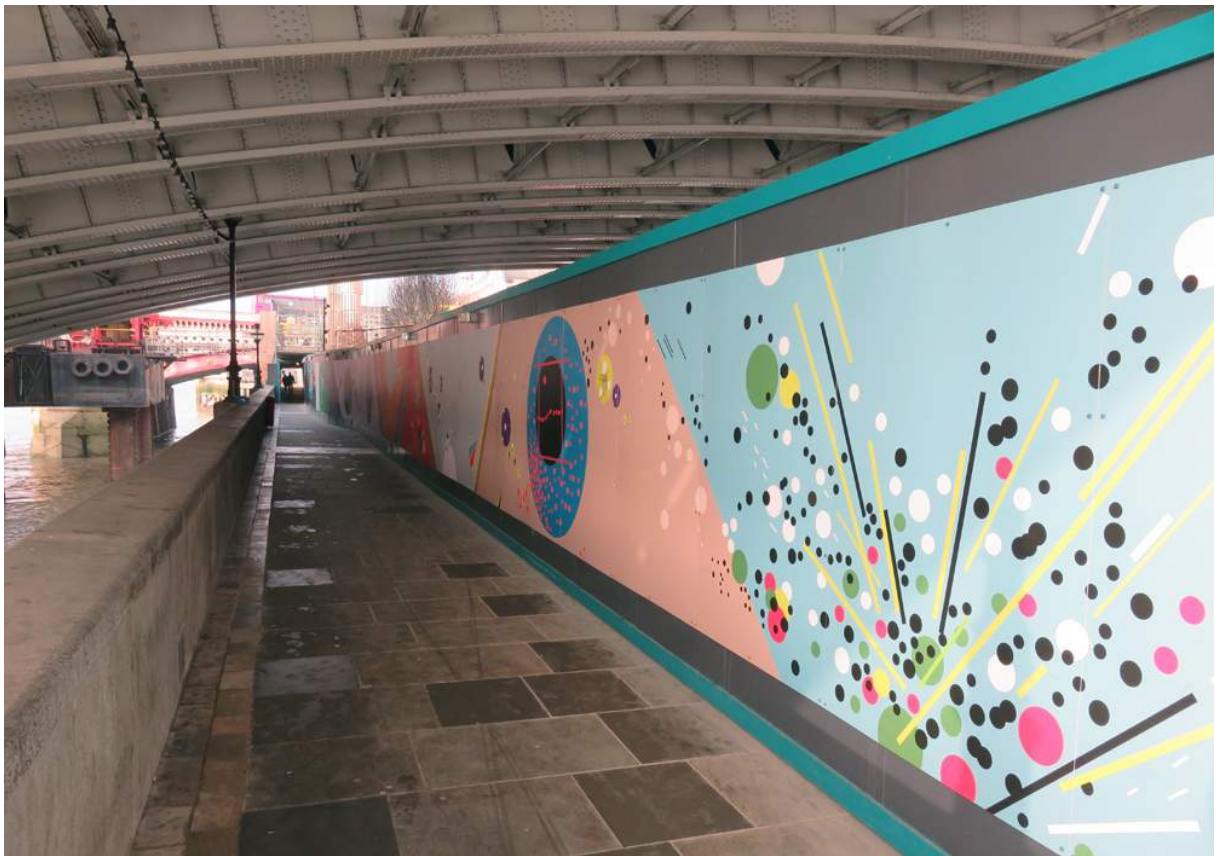
tunnel/map/draw installed on the hoarding at Blackfriars Bridge Foreshore. Photo: Bridget Sawyers
