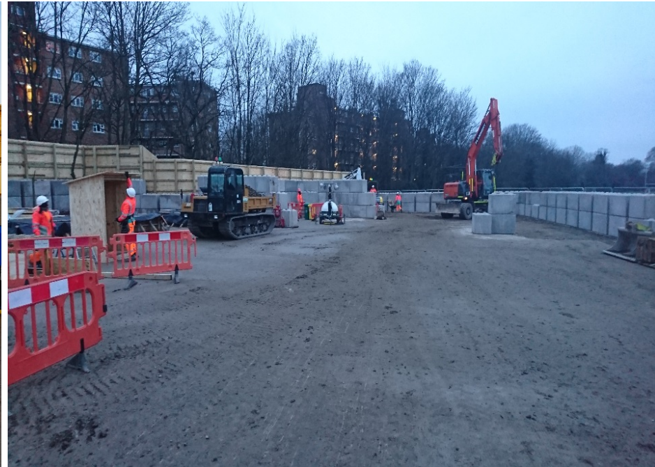
Site set up – welfare, storage, pedestrian routes
