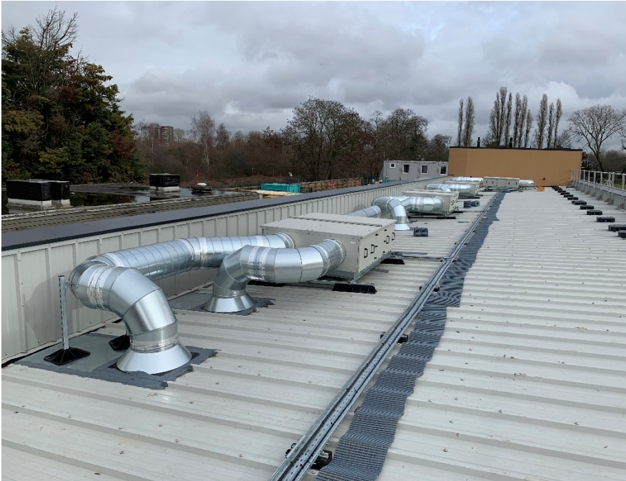
Ventilation on roof
