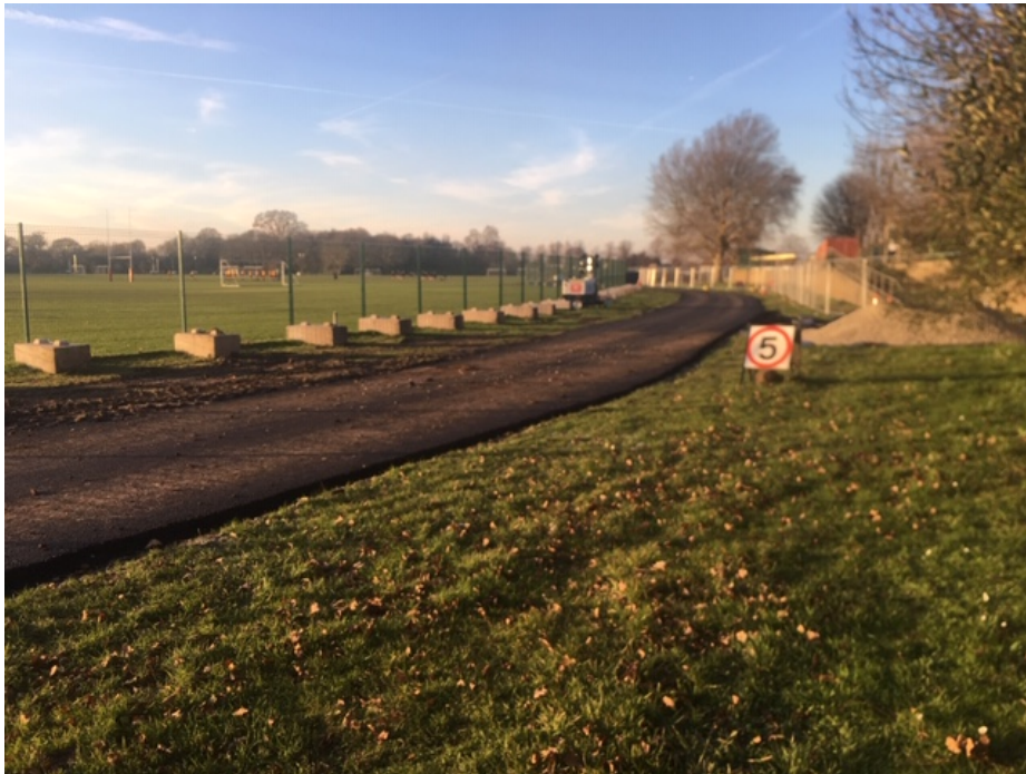
Temporary access road
