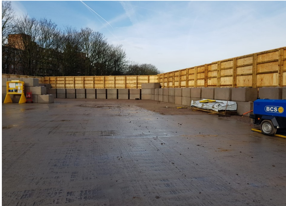
Establishment of the site perimeter security fencing
