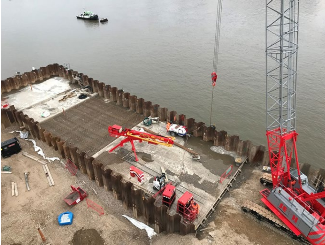
Muck Bin slab cast on 3 January
