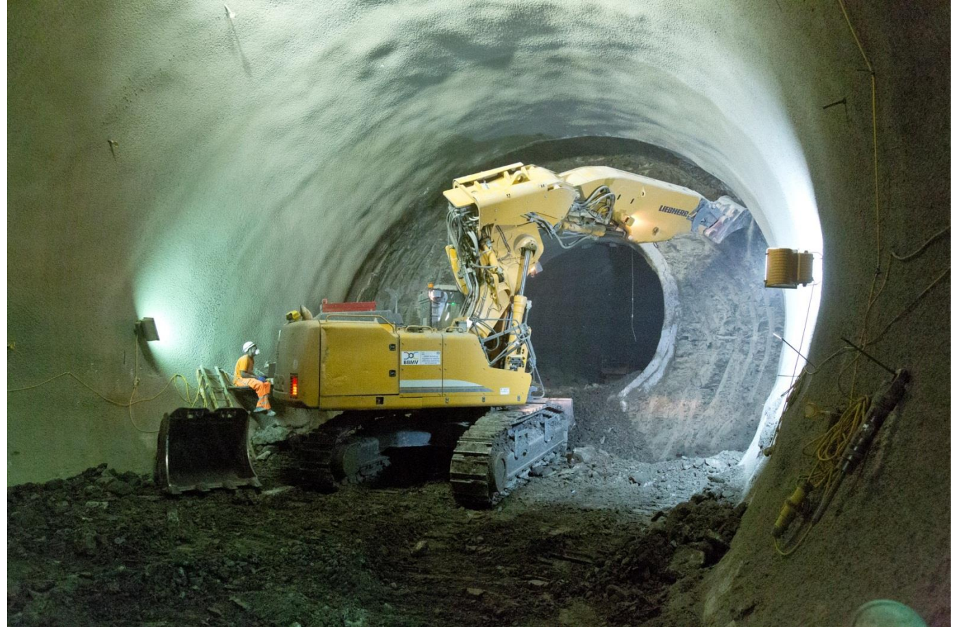
Example of an adit being constructed
