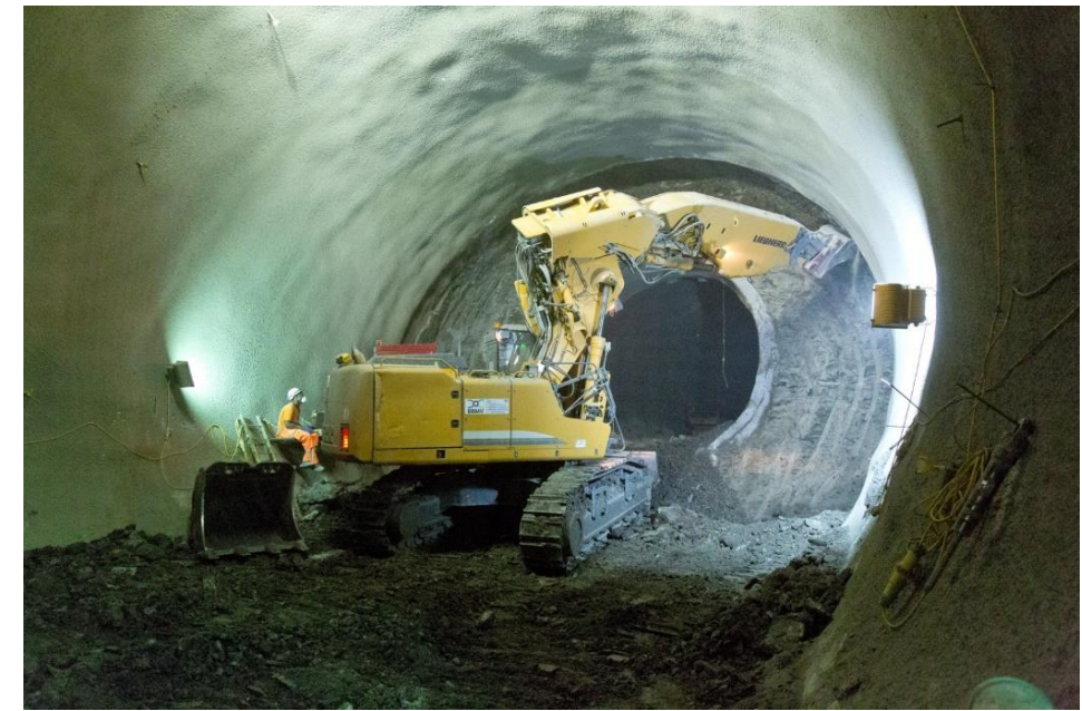
Pictured top right is an example of a tunnel adit being constructed
