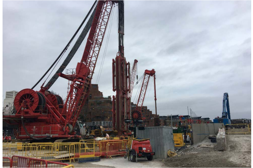
Shaft wall panel excavation
