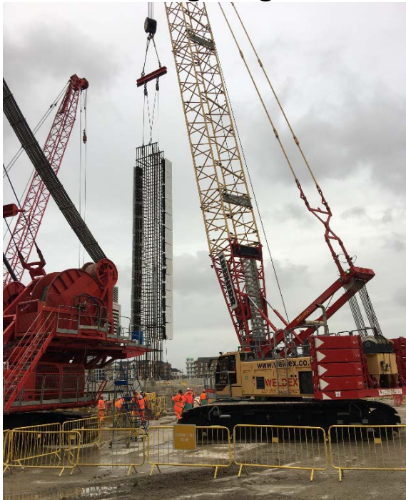
Installing cages
