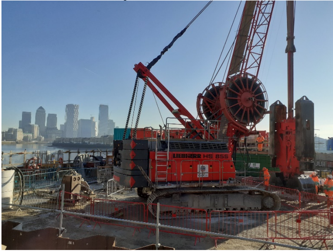
River wall panel excavation
