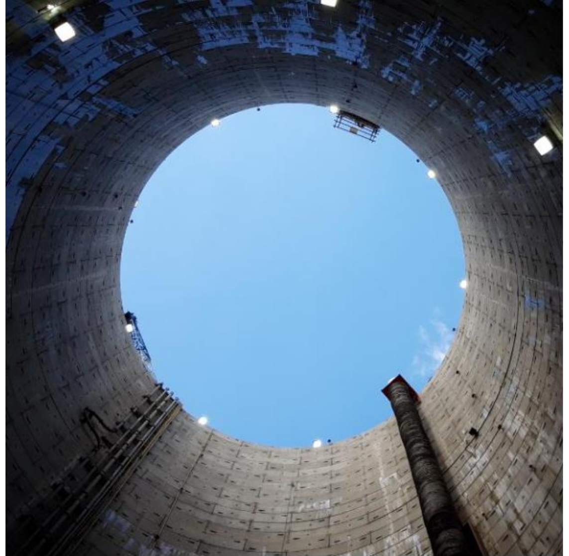
Combined sewer outlet (CSO) shaft
