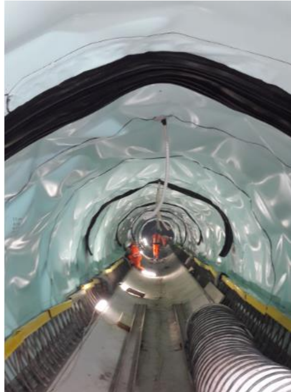
Connection culvert waterproofing
