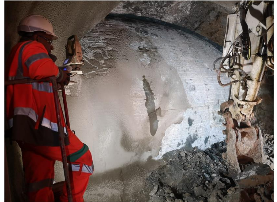
Connection tunnel – reached outer lining of eastbound main tunnel
