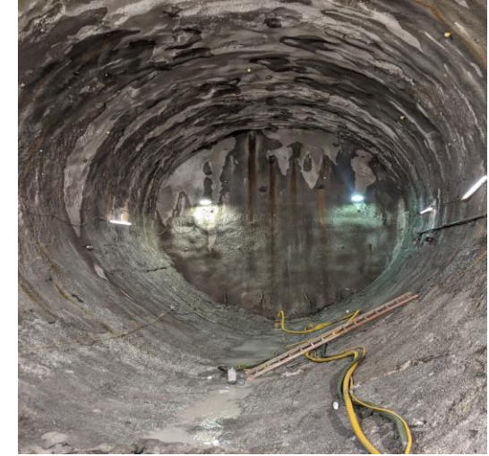
An example of a tunnel adit being constructed
