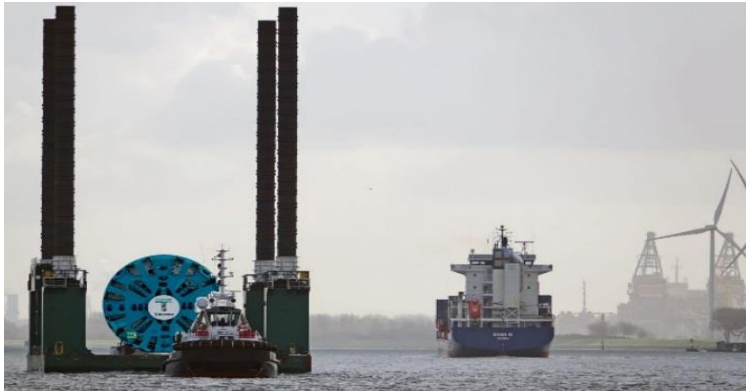
780T TBM Shield on 100T frame delivered by barge
