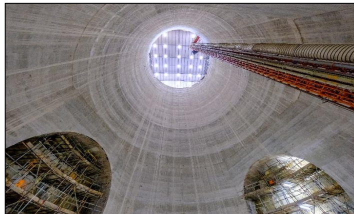
Lower TBM Shield on frame 60m down to the pit bottom
