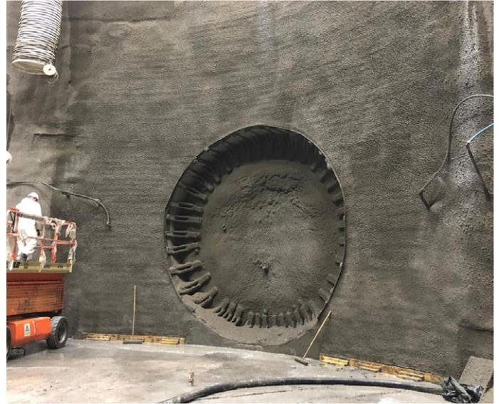
Meanwhile, at Heathwall, the site team has completed the spraying of the portal at the base of the CSO shaft. This marks the conclusion of the primary lining, base slab and portal works in this particular shaft, which is a huge milestone to reach amid challenging working conditions.
