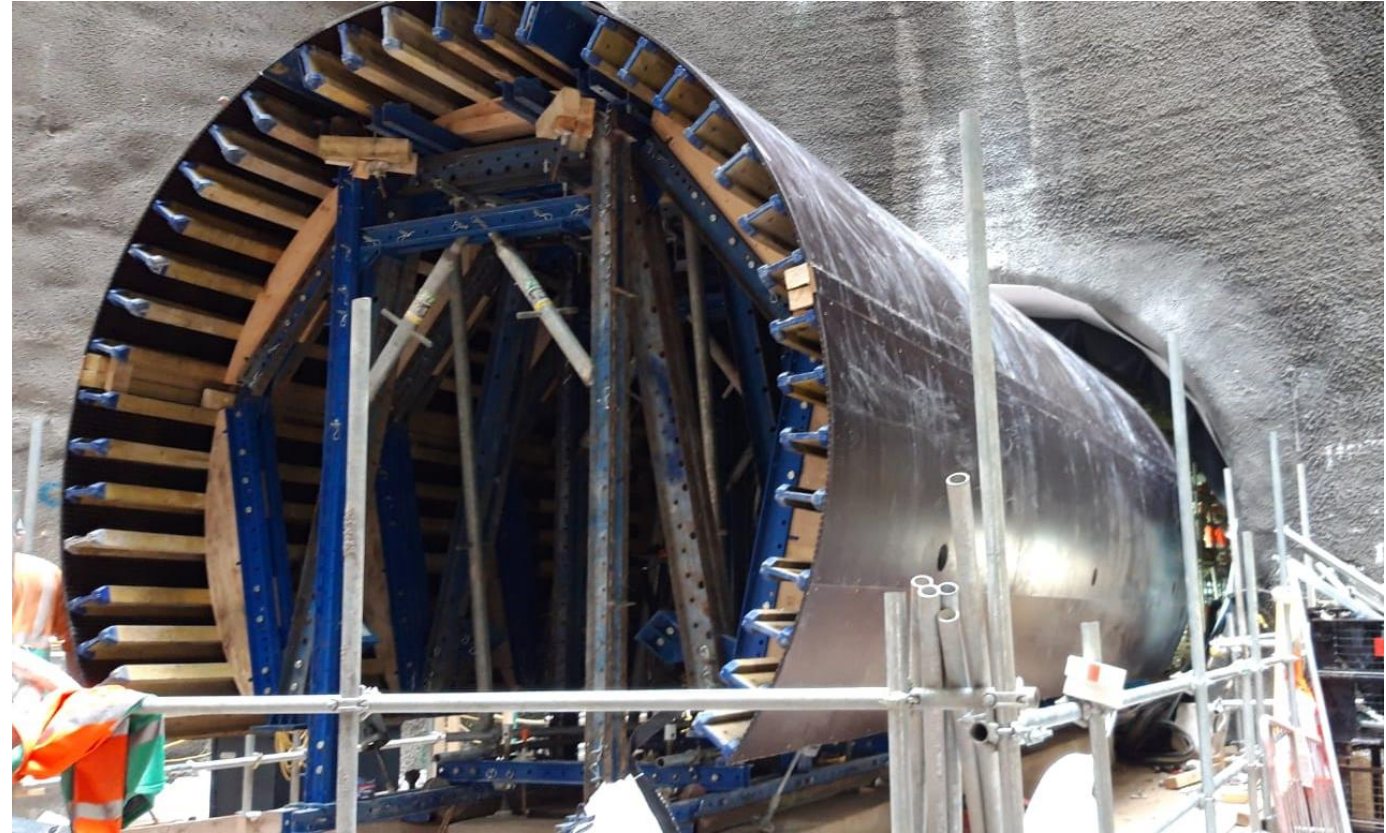
Connection culvert - secondary lining shutter
