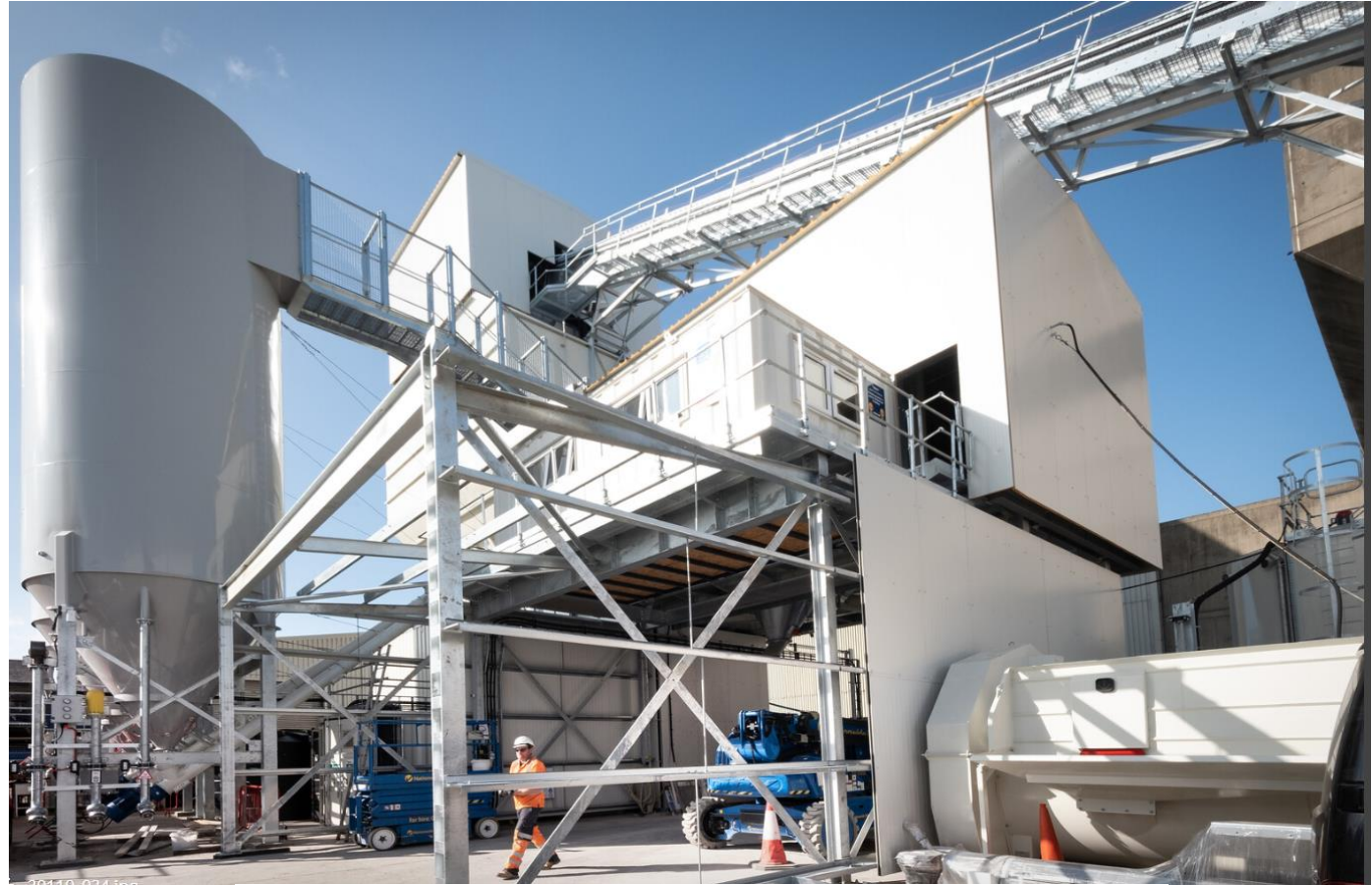
Secondary Lining Concrete batching plant acoustically clad
