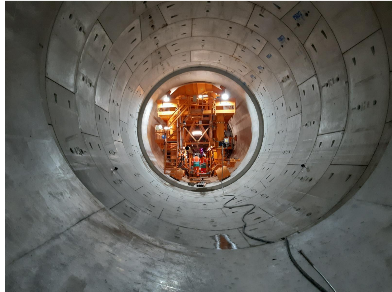
Secondary Lining - Concrete Shutter
