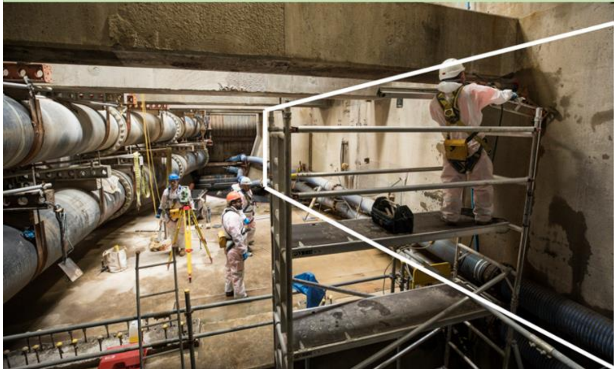
Inlet Channel – Existing wall to be cut out and new wall cast
