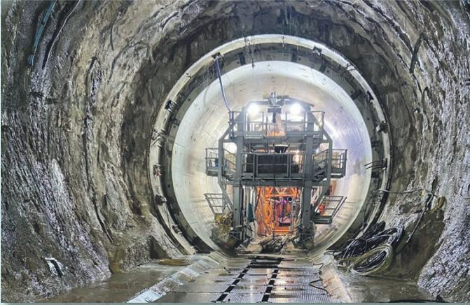
The secondary lining is needed to add extra strength to the tunnels, and will create a smooth surface over which the sewage can flow once the tunnel is operational in 2025.
