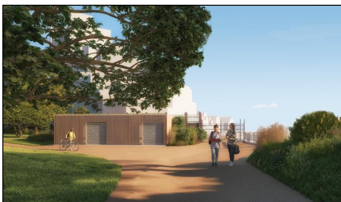
Electrical and mechanical kiosk
