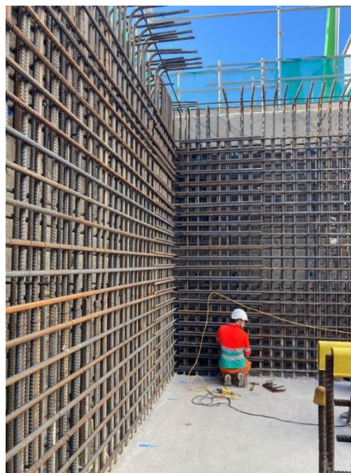
Photograph shows steel reinforcement installed in the Air Treatment Unit
