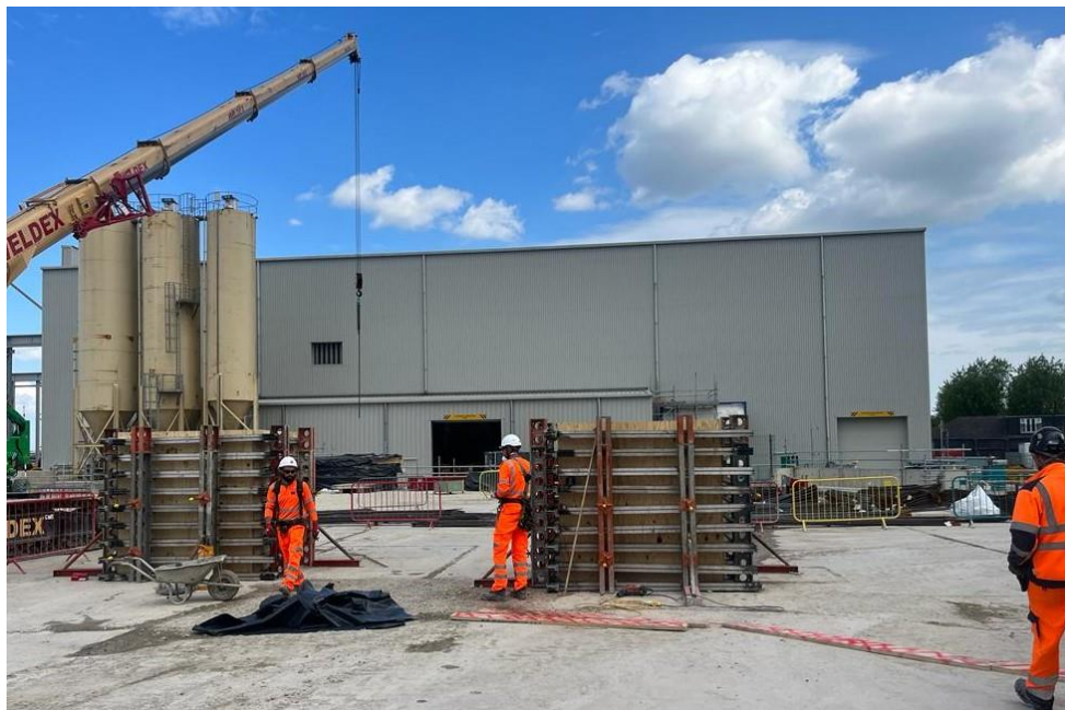
Photograph shows the Chambers Wharf site team installing shutters for pre-cast concrete support blocks
