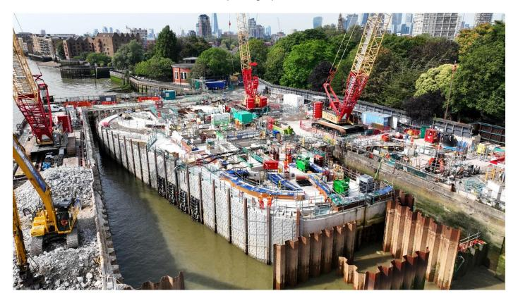
The concrete working platform is being cut into sections, broken up and removed, to be reused as aggregate. We are now using two excavator machines with hydraulic breakers, to speed up the process as they move clockwise around the new, permanent structure.
