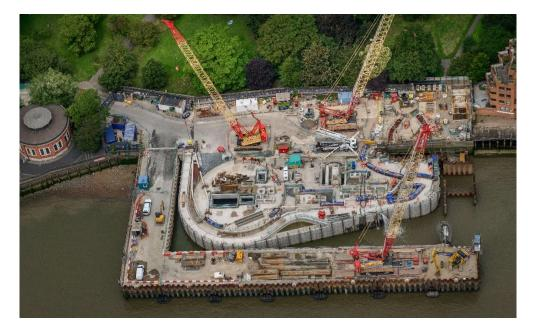
The concrete working platform, which formed the surface of the cofferdam, is being cut into sections, broken up and removed, to be reused as aggregate.
