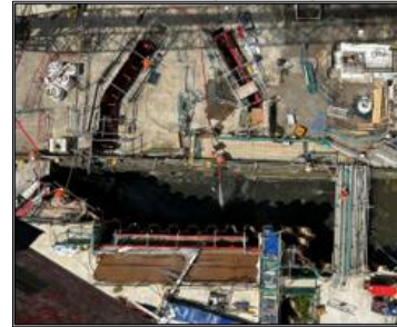
North East Sewer Relief (NESR)
