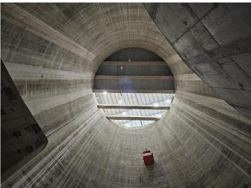
The left image shows steel fixing over the shaft cover slab concrete planks. On the right an upward view from inside the shaft shows the partly completed cover slab.
