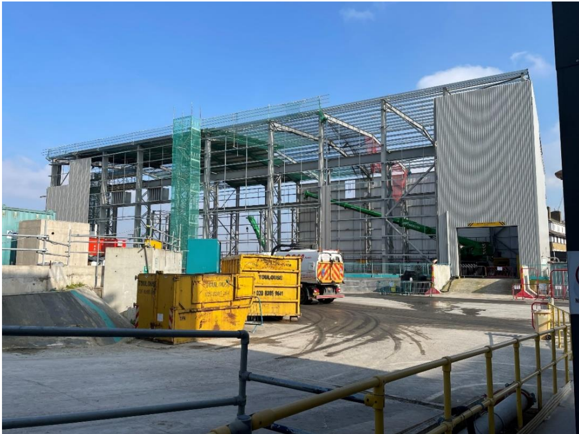
Image showing the partly disassembled noise enclosure
