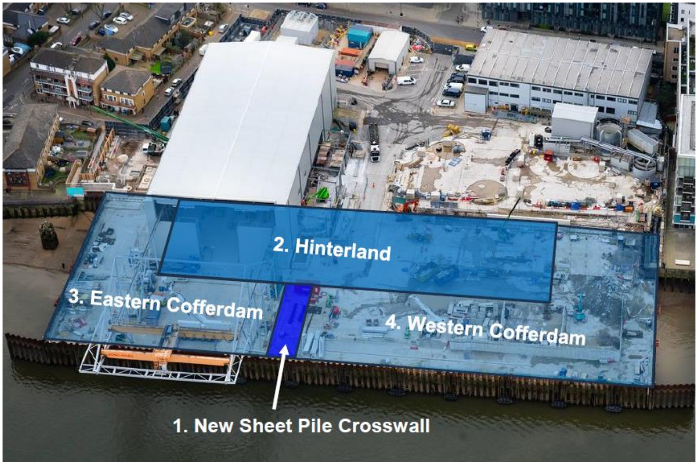
Image showing the four main stages of cofferdam removal
