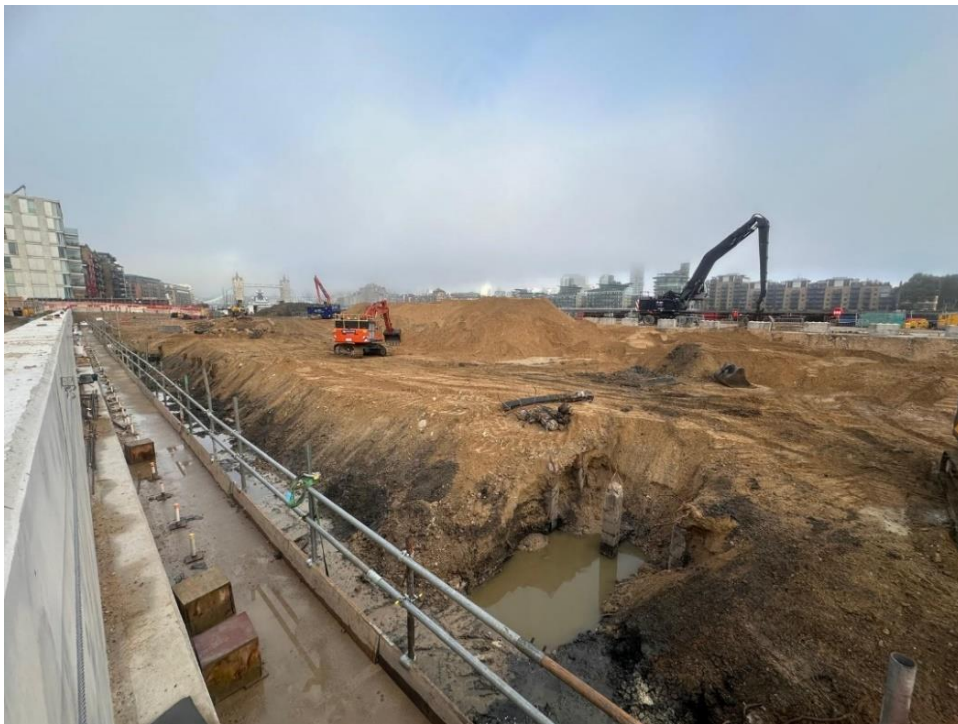
Hinterland excavation & stockpiling, ready for removal
