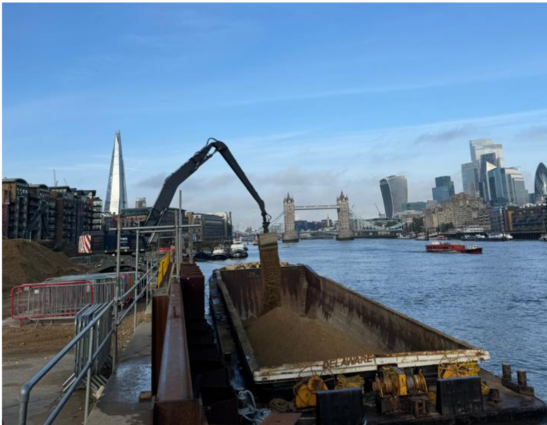
Loading fill material into a barge before it is removed from the site
