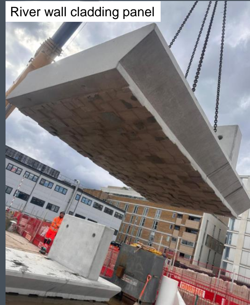
River wall cladding yard inspection
