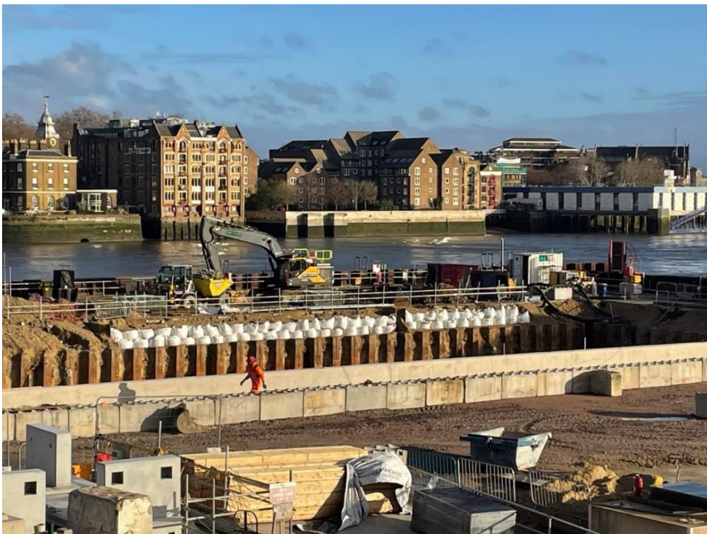
Photograph shows the continued progress of cofferdam removal, looking north-east
