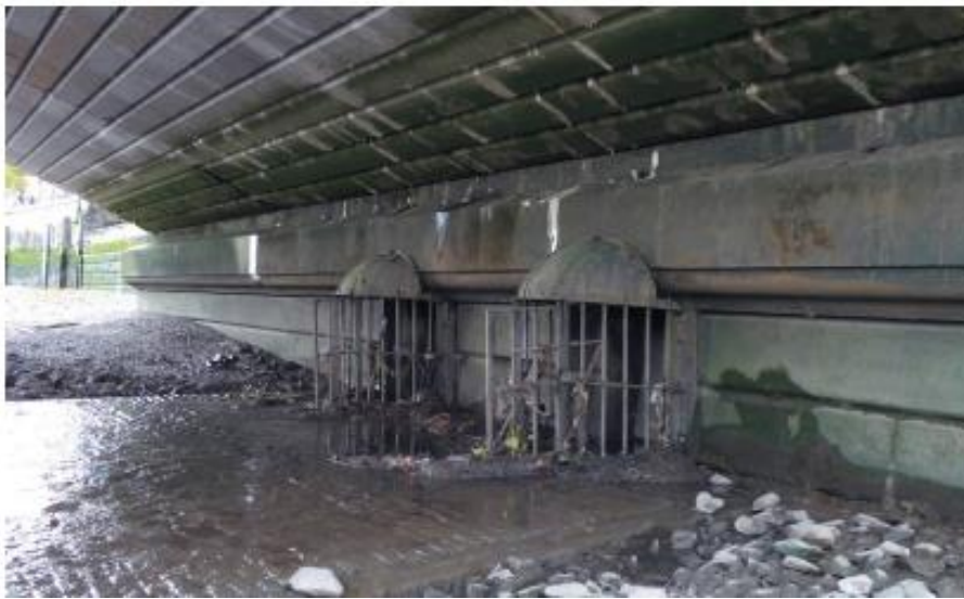
Figure 2-1 Putney Bridge CSO outfall
