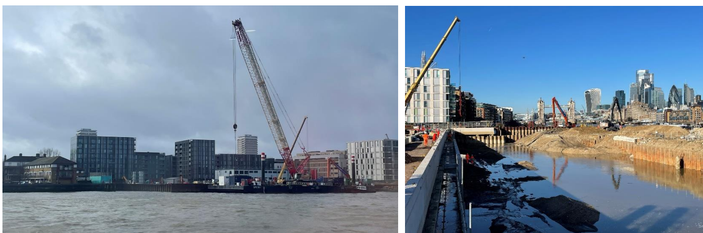
Photographs show the site from the river and cofferdam excavation
