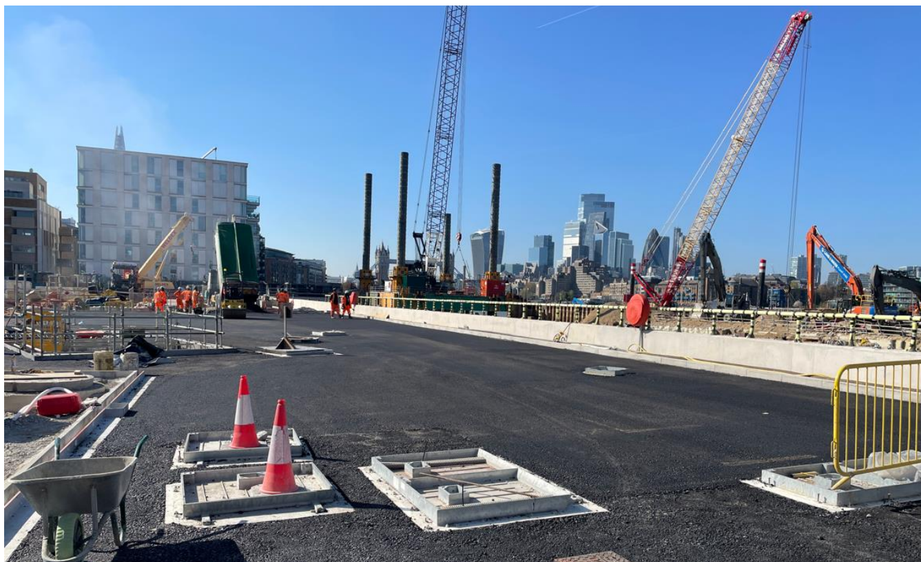
Photograph of the new asphalt placed over the shaft
