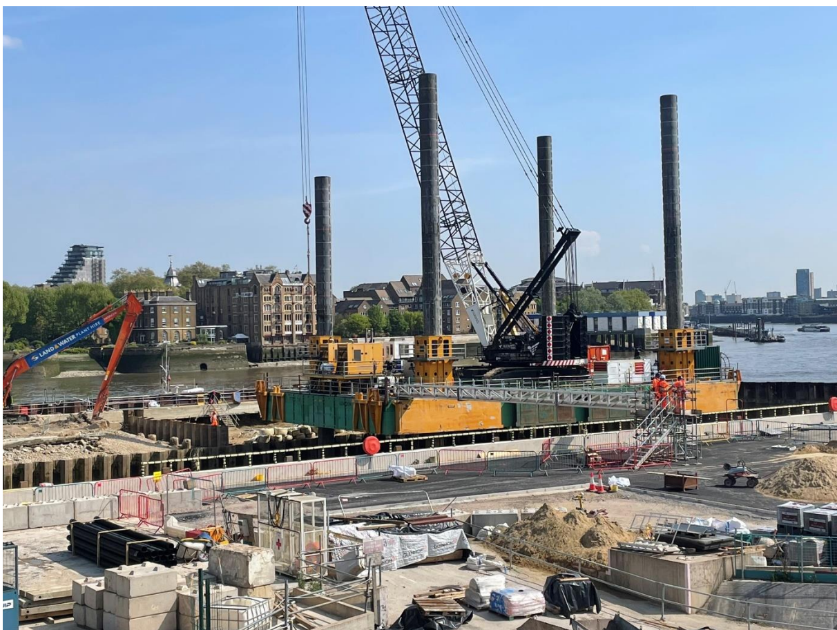
The Jack-Up barge continues to assist operations to remove the cofferdam
