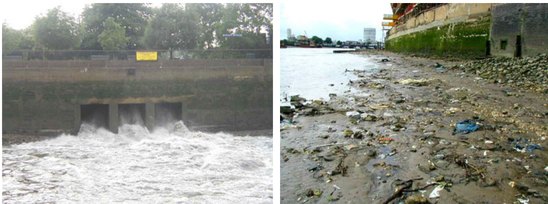
Figures 2 & 3 - Overflows in operation and sewage-derived litter
