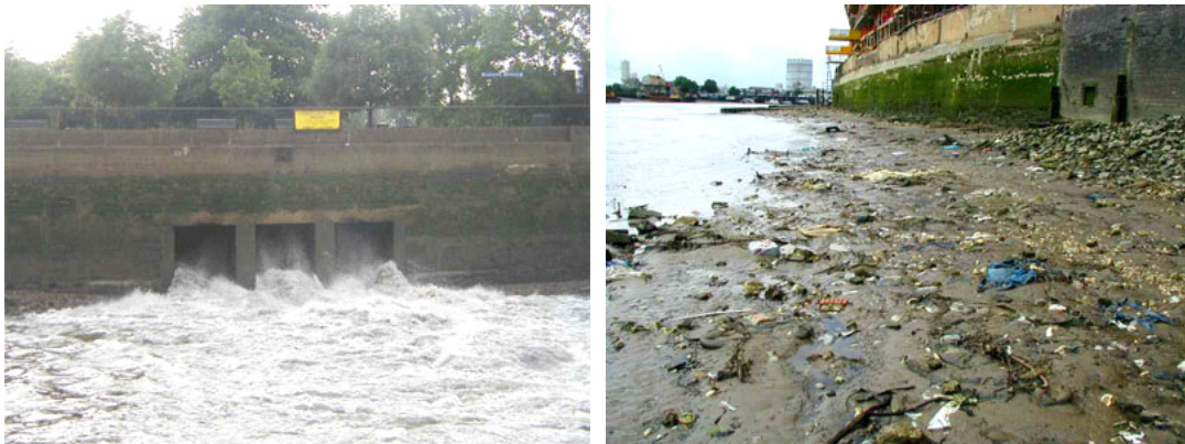
Figure 3 & 4 - Overflows in operation and sewage-derived litter
